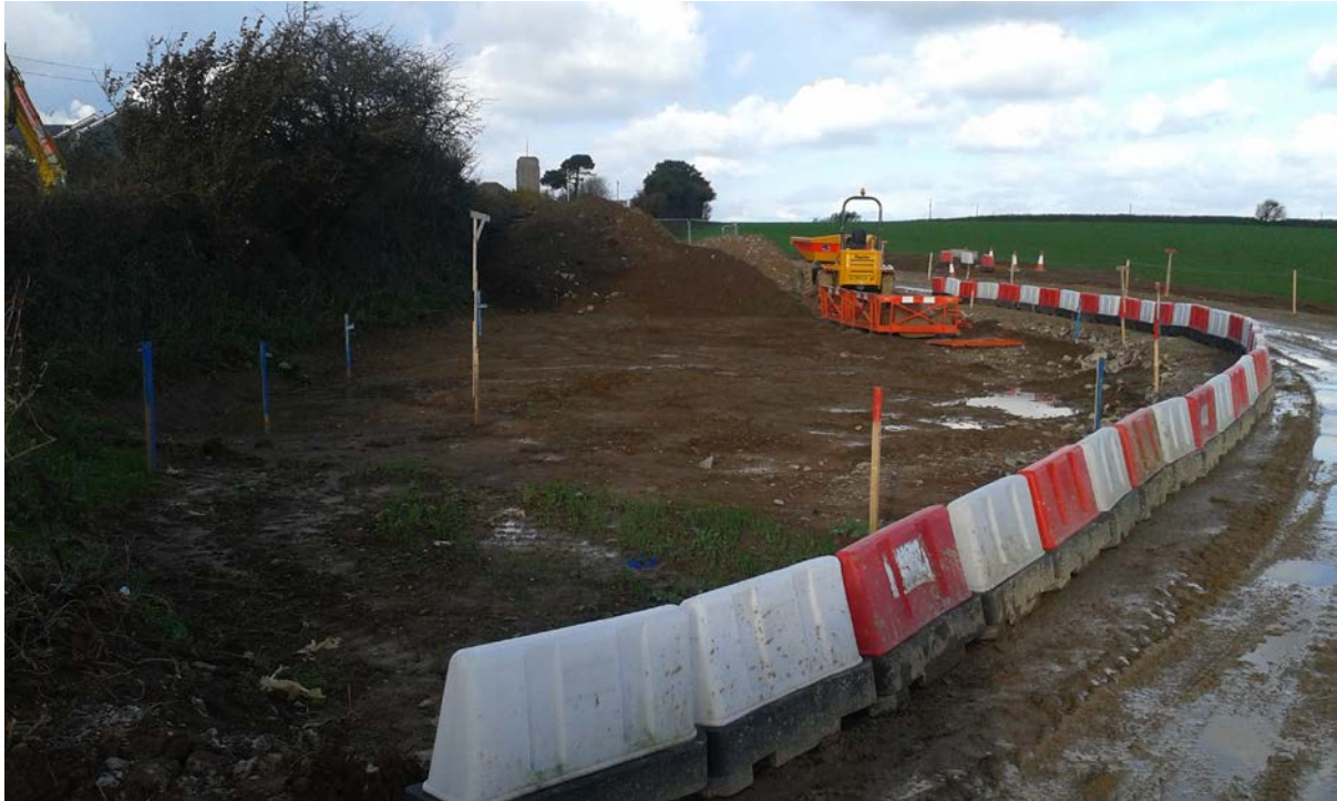
North bound drainage basin construction
