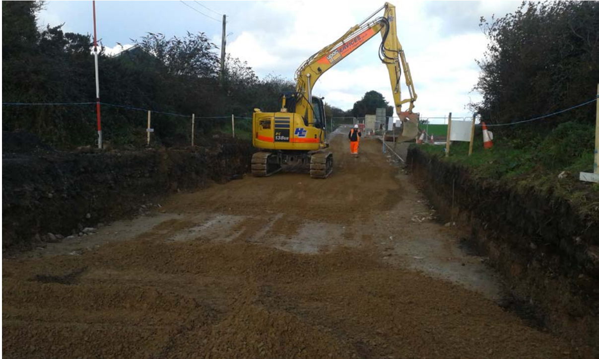
North side road build
