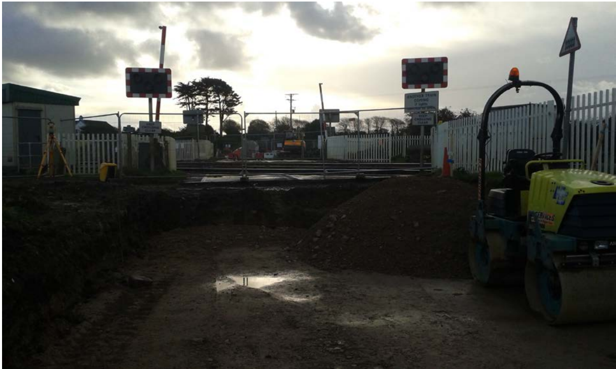
Road construction before level crossing
