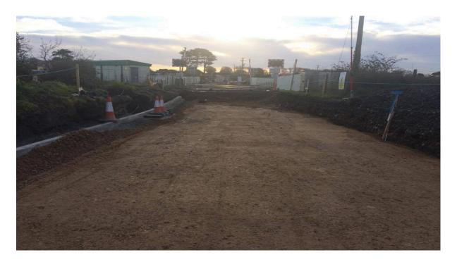
Kerbs and sub base north side of the track looking away from the Level crossing towards the new concrete bellmouth and access track.
