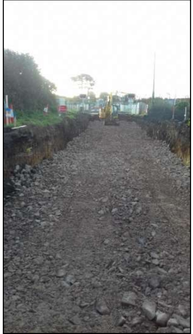
The excavation of the North section is almost complete. Capping stone has been laid ready for compaction
